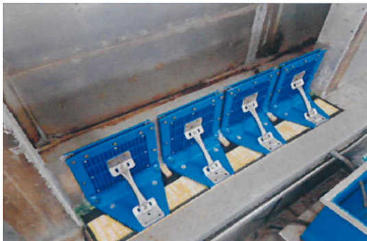
Fig. 7. After test specimen installation
