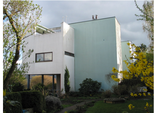
Fig. 8. Back view of Stuttgart house
