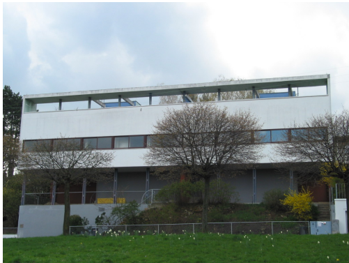
Fig. 7. Front view of Stuttgart house
