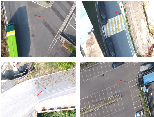
Fig. 12. Check Points of UAV
