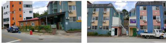
Fig. 14. Utilizing external public space Status in B Zone
