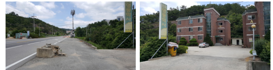
Fig. 3. Status of A Zone Entrance
