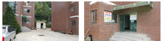
Fig. 10. Utilizing external public space Status in A Zone
