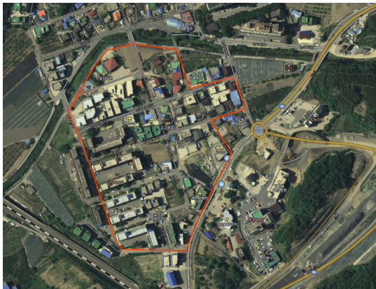
Fig. 6. Status of exterior Space in C Zone
