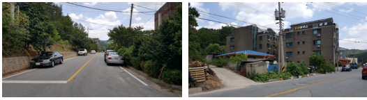
Fig. 5. Status of B Zone Entrance
