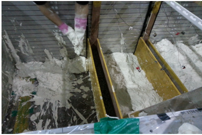
(a) clay and crushed stone foundation construction
