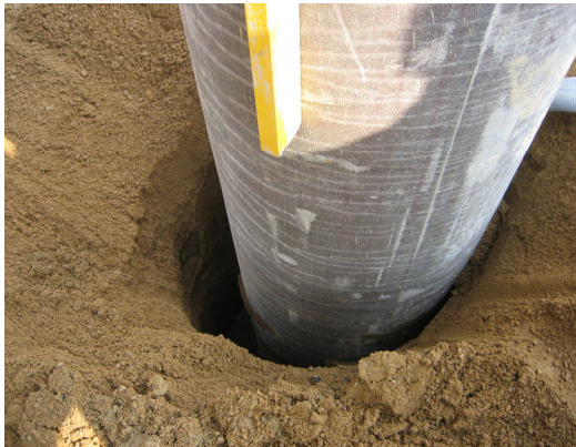
Fig. 5. UΦ4550 pile construction foreground
