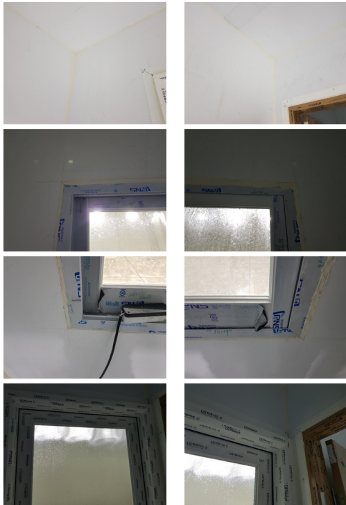
Fig. 14. Result of Rainfall test
