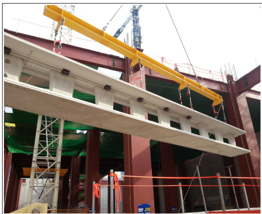
Fig. 5. MDW unloading and installation
