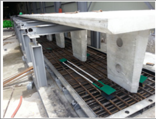
Fig. 4. MDW Reinforcement and formwork installation
