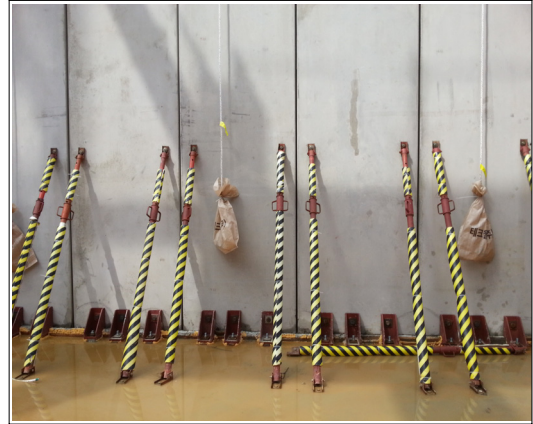
Fig. 6. MDW support and base anchor installation after MDW assembly
