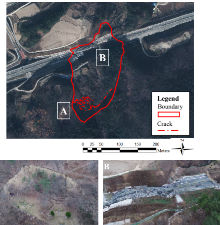
Fig. 5. Results of slow-moving landslide crack extraction at the study site
