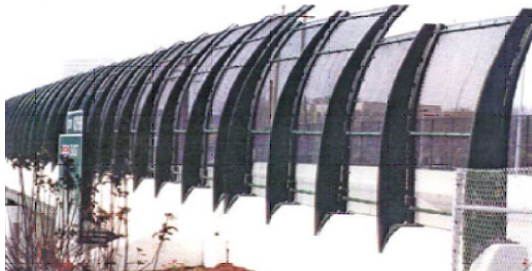
Fig. 6. Spring street bridge
