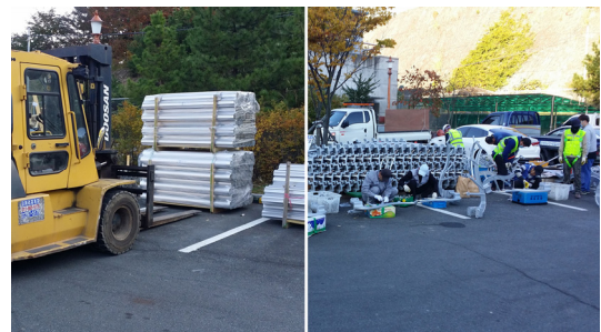
Fig. 17. Rollinder System before construction preliminary work
