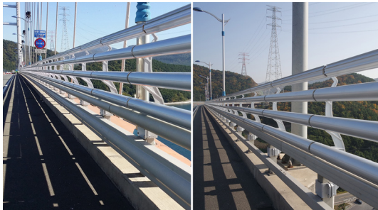
Fig. 19. Rollinder System completion of construction
