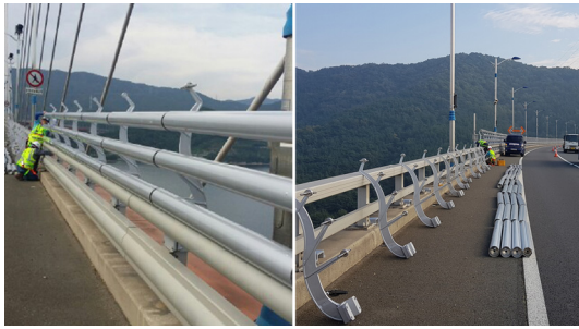
Fig. 18. Rollinder System under construction
