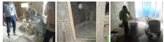
Fig. 9. Waterproofing mortar Mixed
