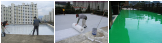
Fig. 6. Liquid-applied membrane waterproofing construction Method
