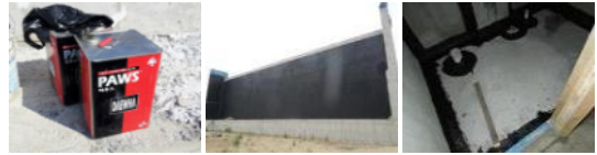
Fig. 7. Asphalt Waterproof Applying Area
