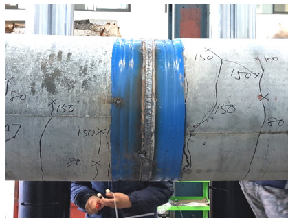
Fig. 10. Concrete cracks in sample RC500-F-J after the bending test
