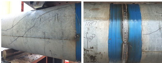
Fig. 13. Concrete cracks in sample RC500-S-J
