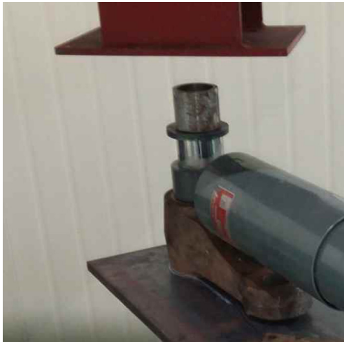
Fig. 8. Assembly of new elastic joint
