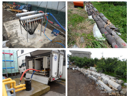
Fig. 1. Photograph of Jeju type GHXs and rock constructions
