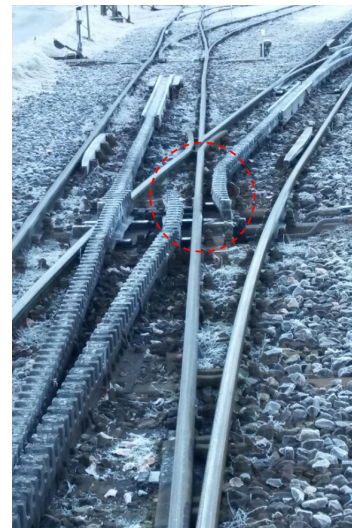
Fig. 3. Conventional branches of rack track
