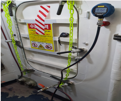
Fig. 3. Established Compartments Leak Test Method
