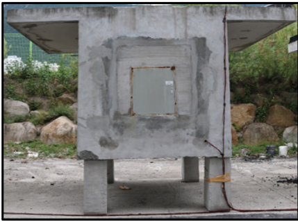
Fig. 1. Front photo of the bridge specimen
