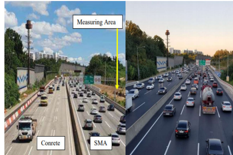
Fig. 1. Before(left) and After(right) Applying Low Noise Pavement on the Test Section
