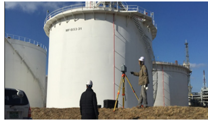
Fig. 2. Oil Storage tank
