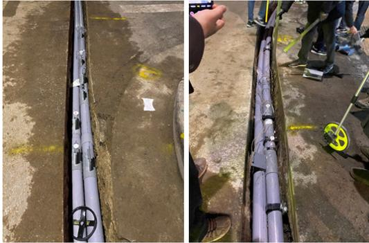
Fig. 6. Sensor installation on Seoul Yang-cheon district
