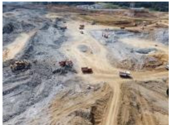
Fig. 3. Background condition of construction site
