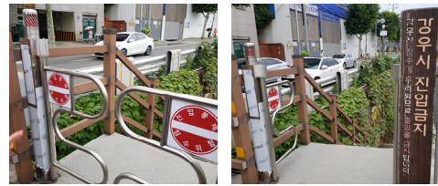
Fig. 11. River entrance blocking facility
