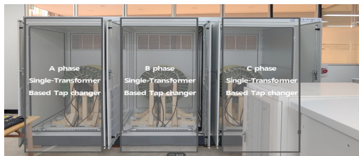
Fig. 9. 30kW scaled Artificial Test Facility
