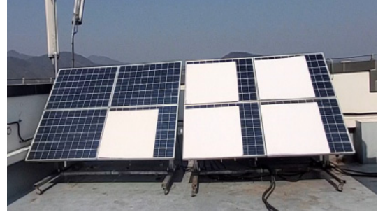
Fig. 10. Shading conditions of PV string
