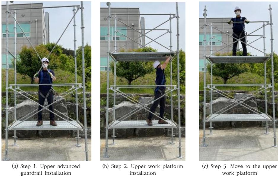
Fig. 4. Installation of Advanced Guardrail
