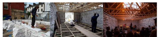
Fig. 13. The Construction Process of OTO Project[37]
