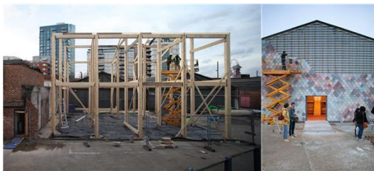
Fig. 11. The Construction Process of Yardhouse ( https://99percentinvisible.org/episode/instant-gramification )
