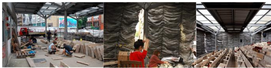
Fig. 14. The Construction Process of Cineroleum ( https://www.archdaily.com/777156/the-cineroleum-assemble )
