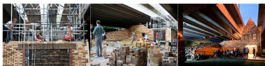
Fig. 15. The Construction Process of Folly For A Flyover[37]
