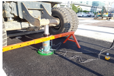
Fig. 5. Plate Loading Test
