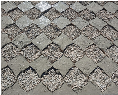
Fig. 3. Geocells filled with cement and aggregates
