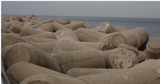
Fig. 2. Panoramic view of rubble mound breakwater armored with tetrapods
