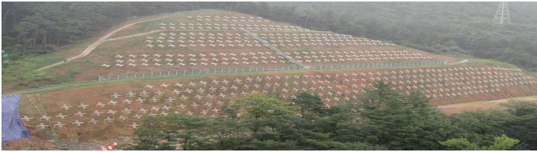
(a) Anchor construction view
