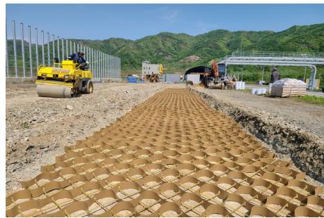
Fig. 5. Placement of Geocell Composite
