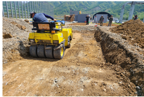
Fig. 4. Preparation for Test Pavement
