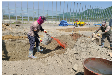
Fig. 6. Mixing of In Site Soil with Binder and Additive
