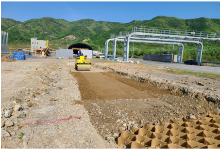
Fig. 7. Placing and Compaction of Solidified Soils
