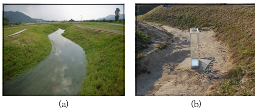
Fig. 1. Experiment channel and bridge pier(REC, Andong) (a) Meandering channel, (b) Small river bridge pier
