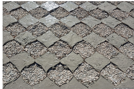
Fig. 4. Geocells filled with cement and aggregates
