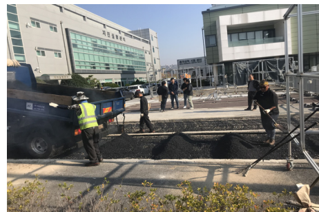
Fig. 5. Placement of porous asphalt mixture
