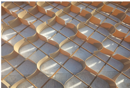
Fig. 2. Geocells reinforced with rebar
