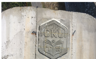
Fig. 11. Final logo clearly engraved on concrete columns
