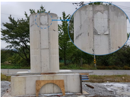
Fig. 10. Attached form liner after removal of concrete form
