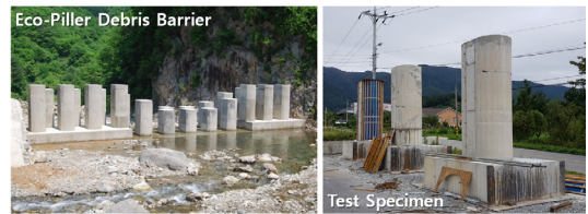
Fig. 5. Eco-pillar debris barrier and test specimen
