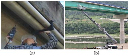
Fig. 1. Anchor bolt insertion drilling work at height for installation of drainage pipes
