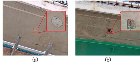
Fig. 5. Drainage facilities installation process after removing the formwork under the bridge
