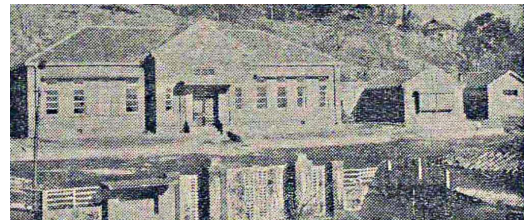
Fig. 11. Front view of Hongwon-gun Office source: [6]
