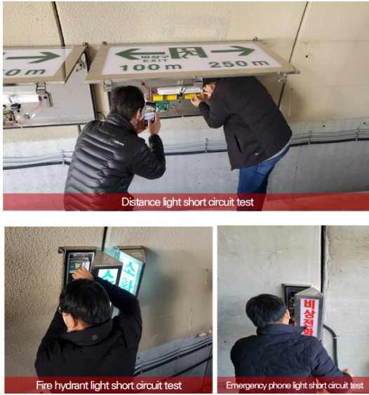
Fig. 11. Short Circuit Test for Spare Power Supply
