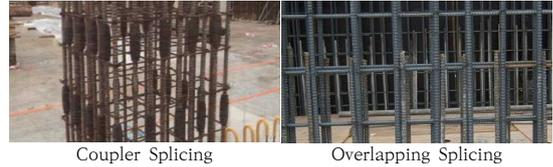
Fig. 7. Reinforcing bar splicing work
