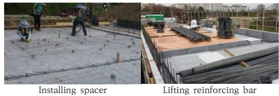
Fig. 8. Reinforcing bar splicing work
