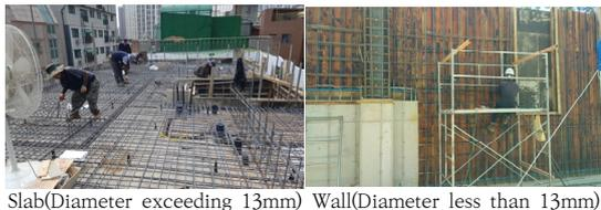
Slab(Diameter exceeding 13mm) Wall(Diameter less than 13mm)
