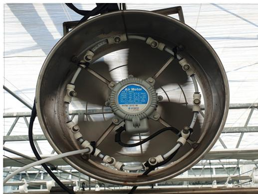
Fig. 2. The combined methods of airflow fan and fog
