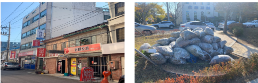
Fig. 3. old buildings and Fig. 4. garbage messing up the city signboards
