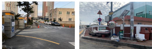
Fig. 7. driveway just outside the gate
