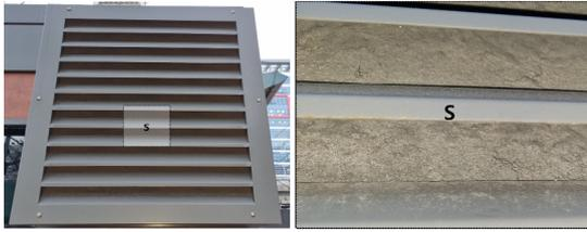
Fig. 1. Blockage of media filter type installed outdoors
