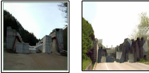
Fig. 7. Rockfall obstacle generated on scale n-2
