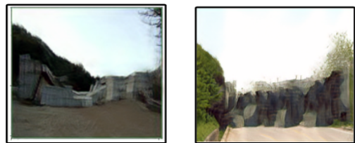
Fig. 6. Rockfall obstacle generated on scale n
