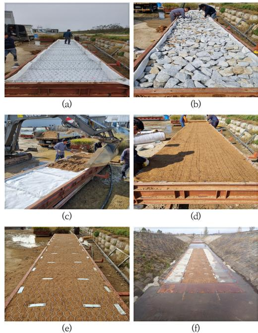
Fig. 4. Installation of the vegetation matrix rip-rap (a) base mesh layer, (b) base gravel filling, (c) Soil filling, (d) vegetation mat covering, (e) finished product, (f) installation
