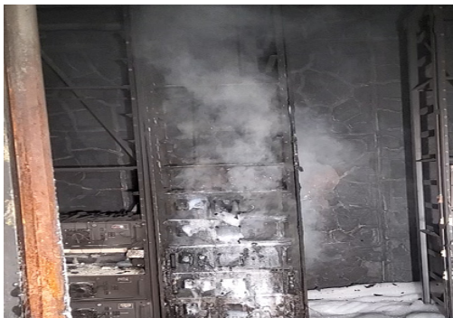
Fig. 11. Complete fire extinguishing in top fire stage of 25kWh Rack
