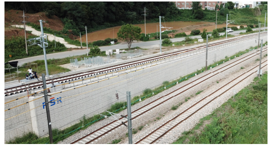
Fig. 4. Construction site of Osong test line
