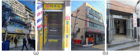
Fig. 4. Elevation and Entrance of Gosiwon in Jong-no 1:2:3:4-ga dong (a) Noah House (b) Sudo Gosiwon
