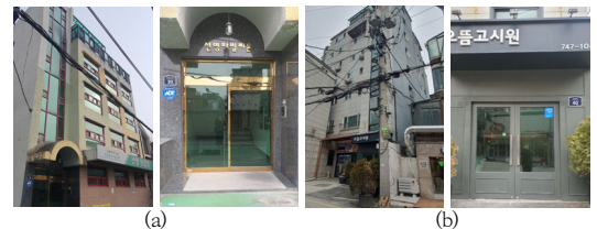
Fig. 6. Elevation and Entrance of Gosiwon in HyeHwa dong (a) Sunmyung Pavilion (b) Euddeum Gosiwon
