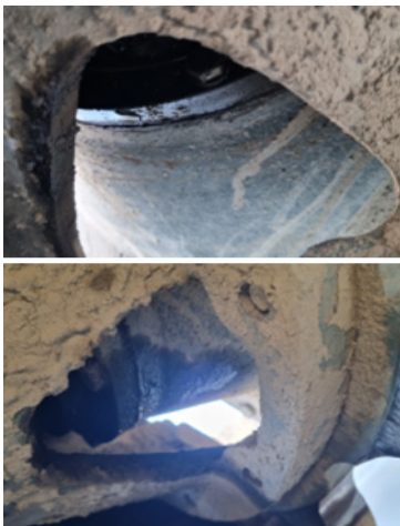
Fig. 8. Leakage of Final Drive Field Verification Test
