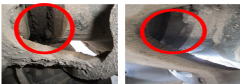
Fig. 1. Leakage of Final Drive
