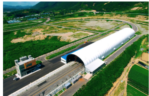
Fig. 5. Adverse Weather Proving Ground: Yeoncheon SOC Research Center
