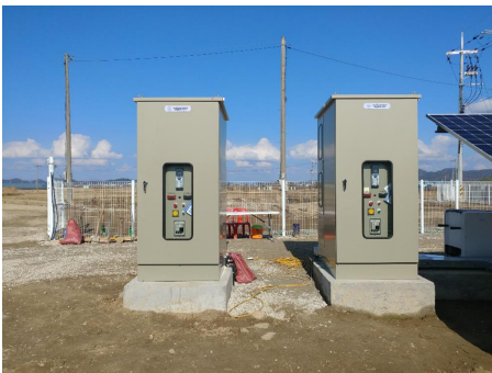
Fig. 4. BIPV GRID Connection System
