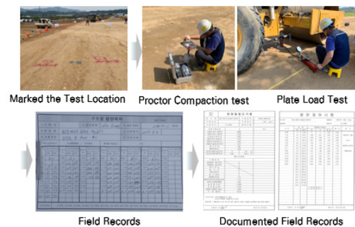
Fig. 1. Conventional compaction quality control Method
