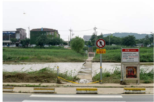
Fig. 4. Safety equipment for Stepping stones in small stream, Cheongju City
